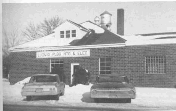
Ludwig's Plumbing, Heating, and Electric on West Main Street.
