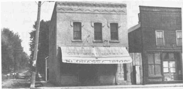
Klobassa Brothers store on the east side of town. Note workers putting in water lines at left.
