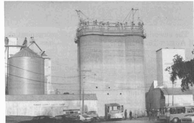
1976—Construction of the cement silos used for grain storage. Capacity of 400,000 bushels.
