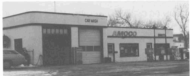
Mort's Amoco and Convenience Store, part of which was the Kinnamon Station, on Busti Avenue.
